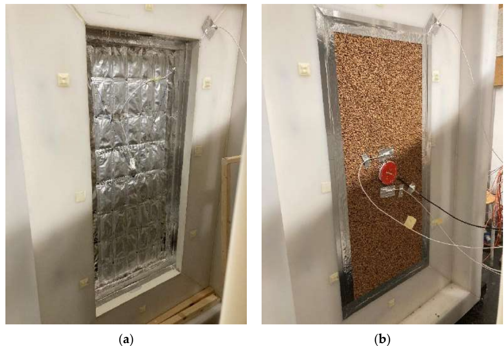
Figure 23. Details of the installation of the PCM sheet inside the SuberWall panel sample (a) and the probes used for the monitoring of the main thermal characteristics (b) by a climatic chamber.
