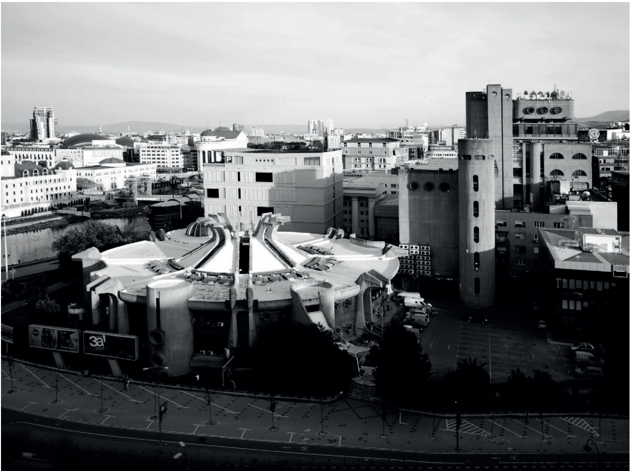
Fig. 4 Janko Konstantinov, Telecommunications Center (1972-1981).
