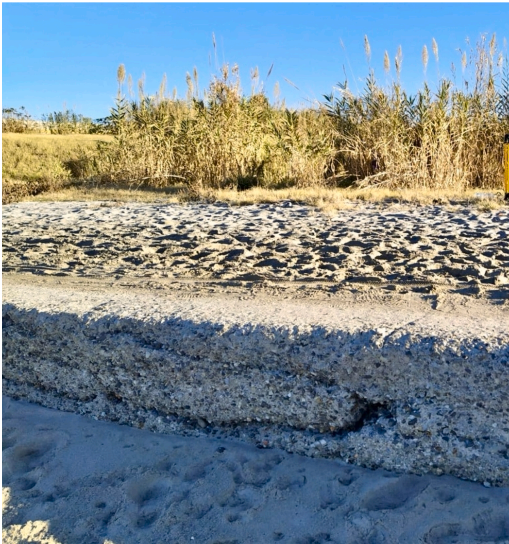
Fig. 10. Fine sediment trapped behind the check dam installed near the mouth of the fiumara Gallico.
