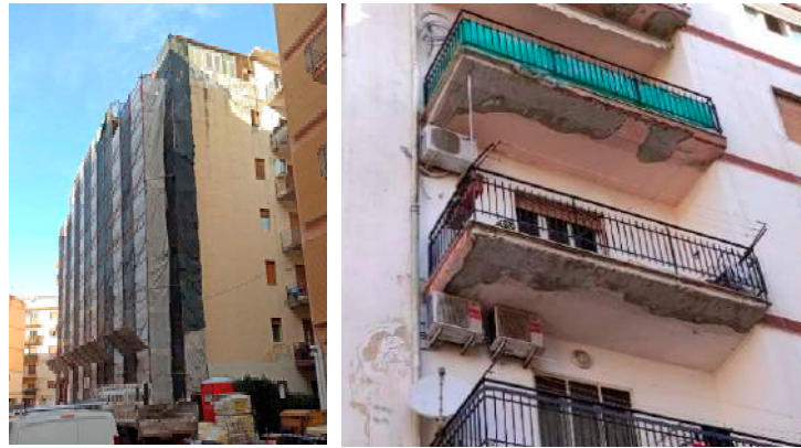
Figure 2. The sample building during the renovation works.
