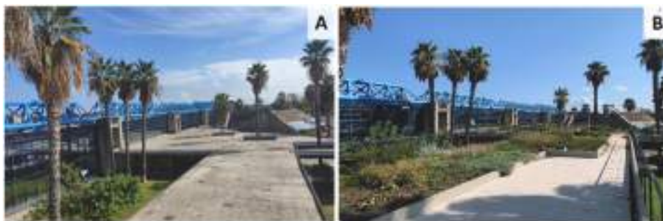
Fig. 2. The roof before green roof installation (A) and after green roof installation (B).
