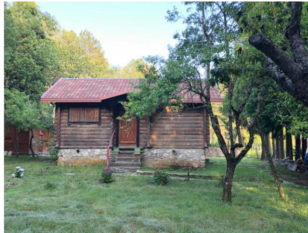
Figure 6. North elevation. Source: Authors.
