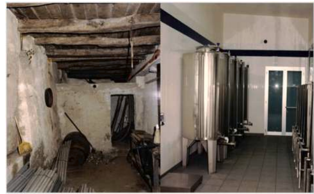
Fig. 2. The Olive Mill (OM) storage room before and after renovation.
