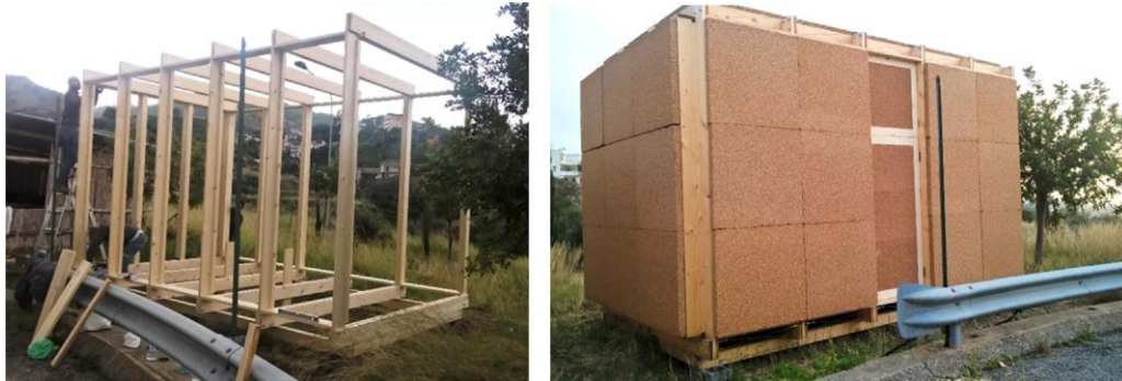
Fig. 6. Construction of the shelter prototype.
