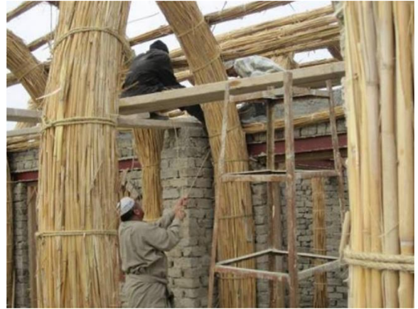
Fig. 2. Arches in giant reed for Mudhif house.
