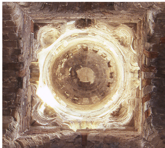
Fig. 13 - Corner squinches. Above left: dome of the church of the Three Saints in San Fratello (Messina), 11th century. Below left: dome of the church of SS. Filippo and Giacomo at the Mareddolce castle in Palermo, XII century. Simple trumpet arches with anteposed arches. Above right: dome of the church of S. Giovanni dei Lebbrosi in Palermo, 11th century. Below right: dome of the church of S. Giovanni degli Eremiti in Palermo, XII century (photo by D. Mediatì).
