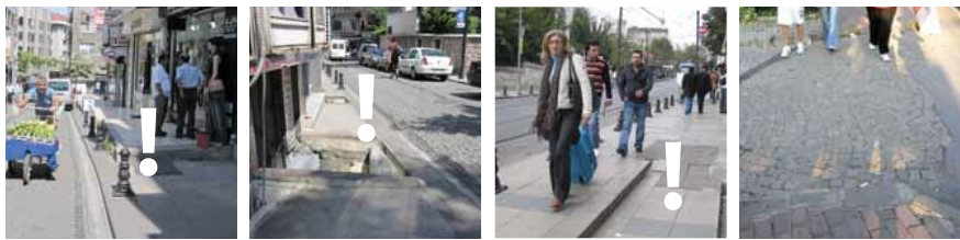
Footways in multiple levels and stairs to basement shops create high risks for tripping. Poor quality paving from unfortunate materials and lack of maintenance create a difficult and an unbecoming patchwork of walking surfaces.
