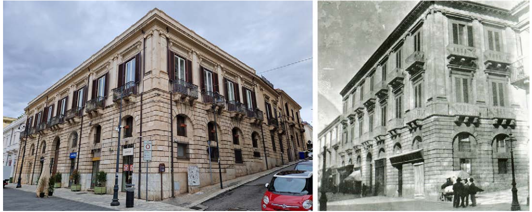
Fig. 2. Melissari-Nesci Palace, Reggio Calabria. Right: photo before the 1908 earthquake. Archivio Nesci, Reggio Calabria [Manfredi 2008, p. 252]. Left: Current state of the palace; the third floor above ground was demolished after the 1908 earthquake.
