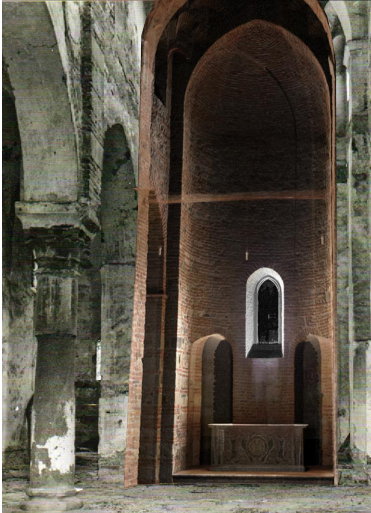
Fig. 6. State of conservation of the church of Saints Peter and Paul, Casalvecchio, 1945, overlapped with the current state (Editing: Marinella Arena).
