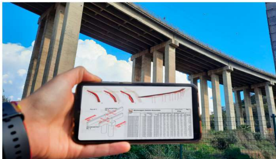
Figure 11. Screenshot example of viewable structural results of the framed viaduct under inspection within the coordinate range.
