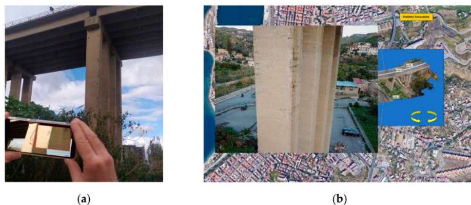
Figure 10. (a) Inspection's detail of the 3D model in AR for the identification of degradation. (b) Visualization of degradation from database image selected from 3D model on the map. The operator can also access it via remote learning on the infrastructure without going to locations.
