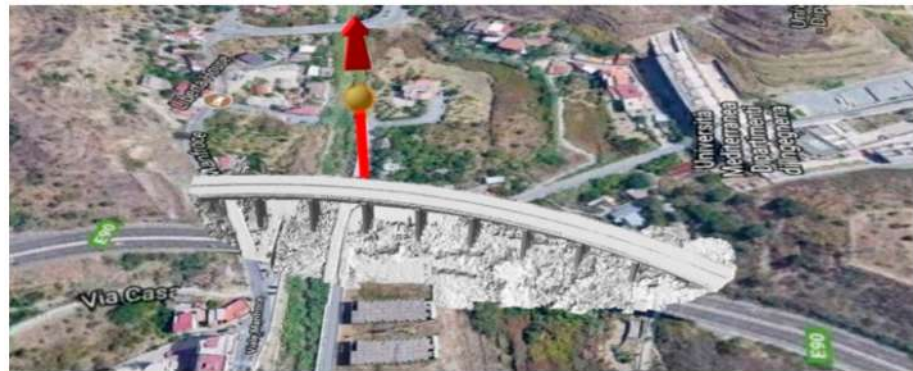
Figure 12. Screenshot extraction of the viaduct deck and its individual constituent elements in Virtual Reality.
