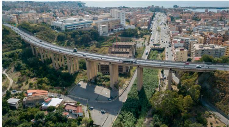
Figure 1. Annunziata Viaduct, Reggio Calabria, Italy.
