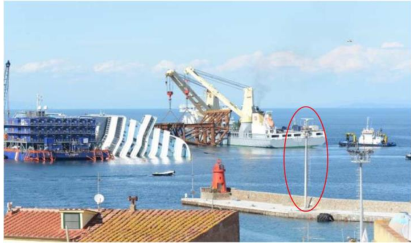
Fig. 4.2 Installation site of the Remocean system indicated by the red circle
