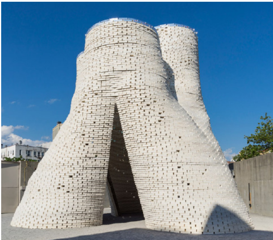
Fig. 10. Hy-Fi, The Organic Mushroom-Brick Tower Opens At MoMA's PS1 Courtyard, 2014. https://www.inexhibit.com/it/case-studies/new-york-hy-fi-installazione-al-moma-ps1/
