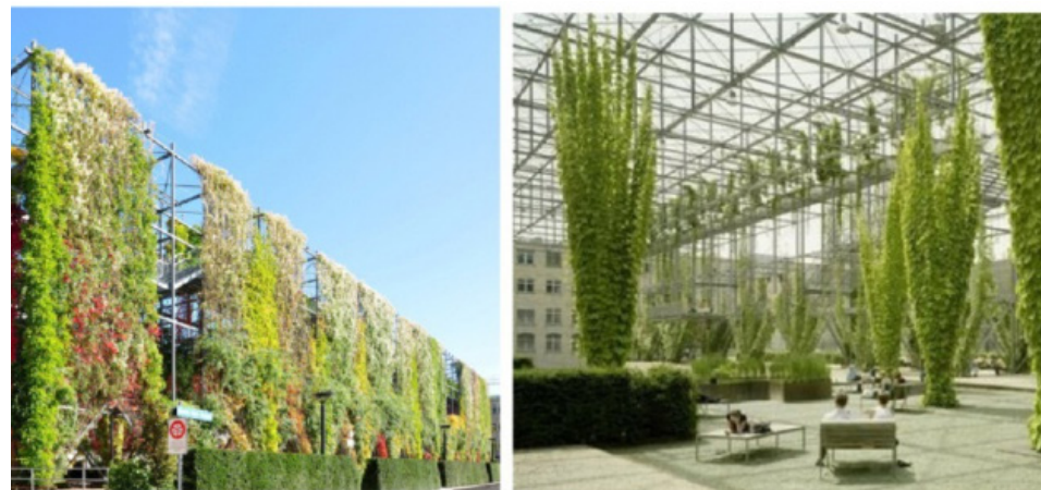
Fig. 2. Grid and Wire-Rope Net Systems, MFO Park Switzerland ( http://commons.wikimedia.org 2013, http://christianbarnardblog.blogspot.com 2013)
