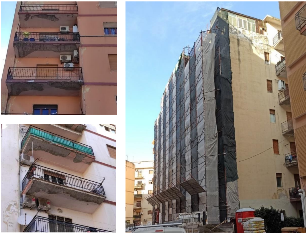
Figure 1. The sample building before and during renovation.
