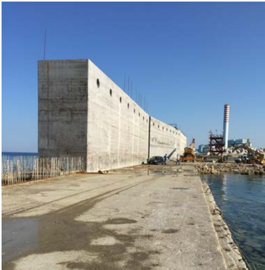
Fig. 1.16: U-OWC breakwater in Civitavecchia, Rome, Italy
