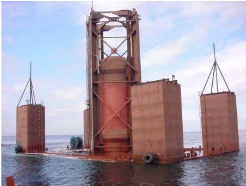
Fig. 1.4: Installation of the AWS pilot plant. From Ref. [3]
