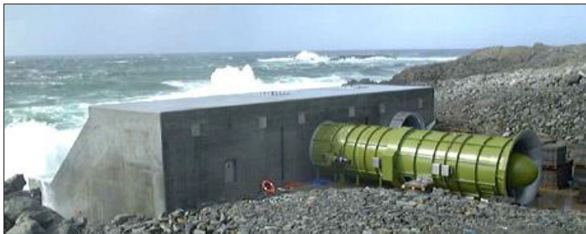
Fig. 1.12: LIMPET OWC wave power plant, Island of Islay, Scotland
