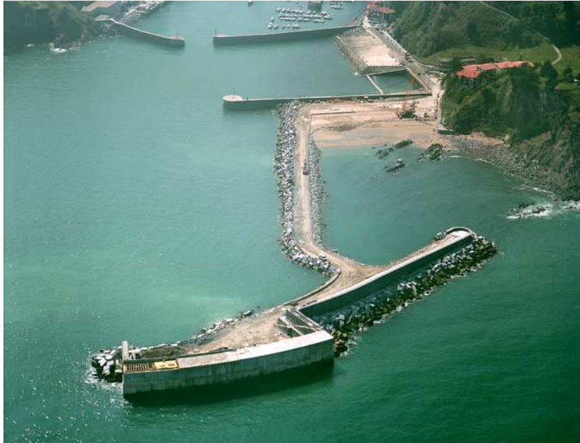
Fig. 1.15: OWC integrated into Mutriku's breakwater, Spain
