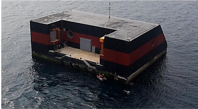
Fig. 1.13: Bottom-standing OWC installed at Yongsoo (Korea)
