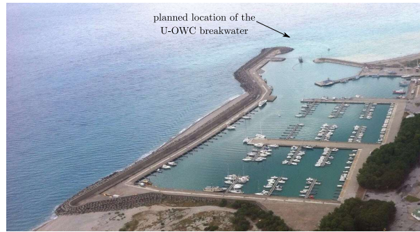
Fig. 3.1: Aerial view of Roccella Jonica marina showing the planned location of the U-OWC breakwater. Courtesy of Marina di Roccella - Porto delle Grazie S.r.l.
