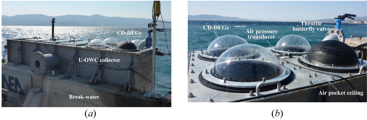
Fig. 4.3: Metallic U-OWC caisson (a) with four CD-DEGs installed on the top of the lateral chamber (b). One of the CD-DEGs was painted black to allow post-processing of the high-speed camera frames.
