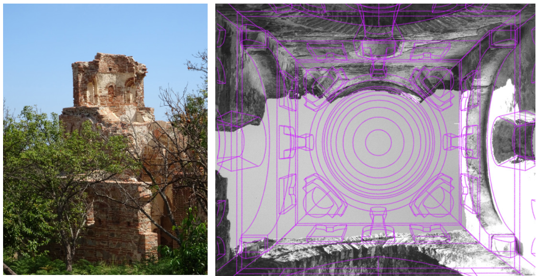
Fig. 7, 8. Santa Maria de' Tridetti, Staiti, 11th-12th century. Left: view of the dome stump from the north-west. Right: hyposcopic view of the dome with superimposed hypothesis of the original configuration. Photo and graphic processing by the author.
