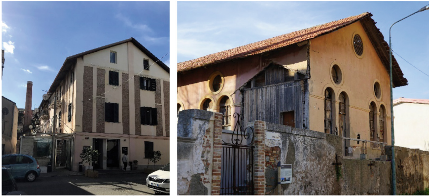
Figs. 3–4. Cannitello (Villa S. Giovanni). On the left, the “Paolo Messina spinning mill” and, in the background, the chimney and the ruin of the “F.lli La Monica” spinning mill; on the right, the “F.lli Cogliandro” spinning mill (photo by the author, 2023).
