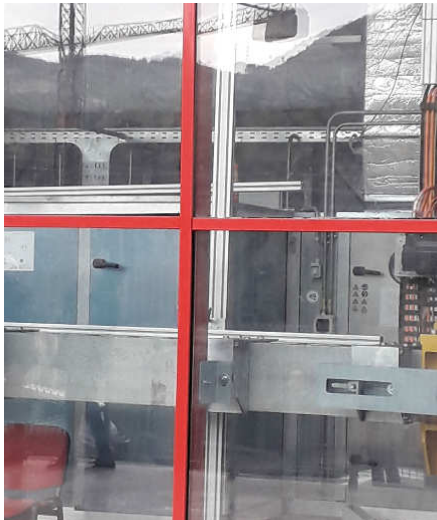
Fig. 29 - Dettaglio mock-up testato in pressione / Detail mock-up tested under pressure (Source: Authors' elaboration).
