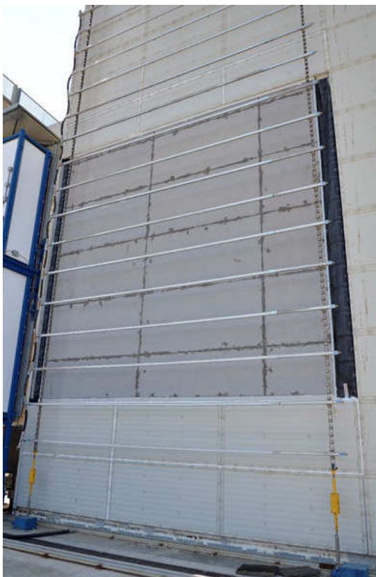
Fig. 30 - Campione sottoposto a prova nell'assetto sperimentale: Full Scale Mock-Up / Sample tested in the experimental setup: Full Scale Mock-Up (Source: Authors' elaboration).
