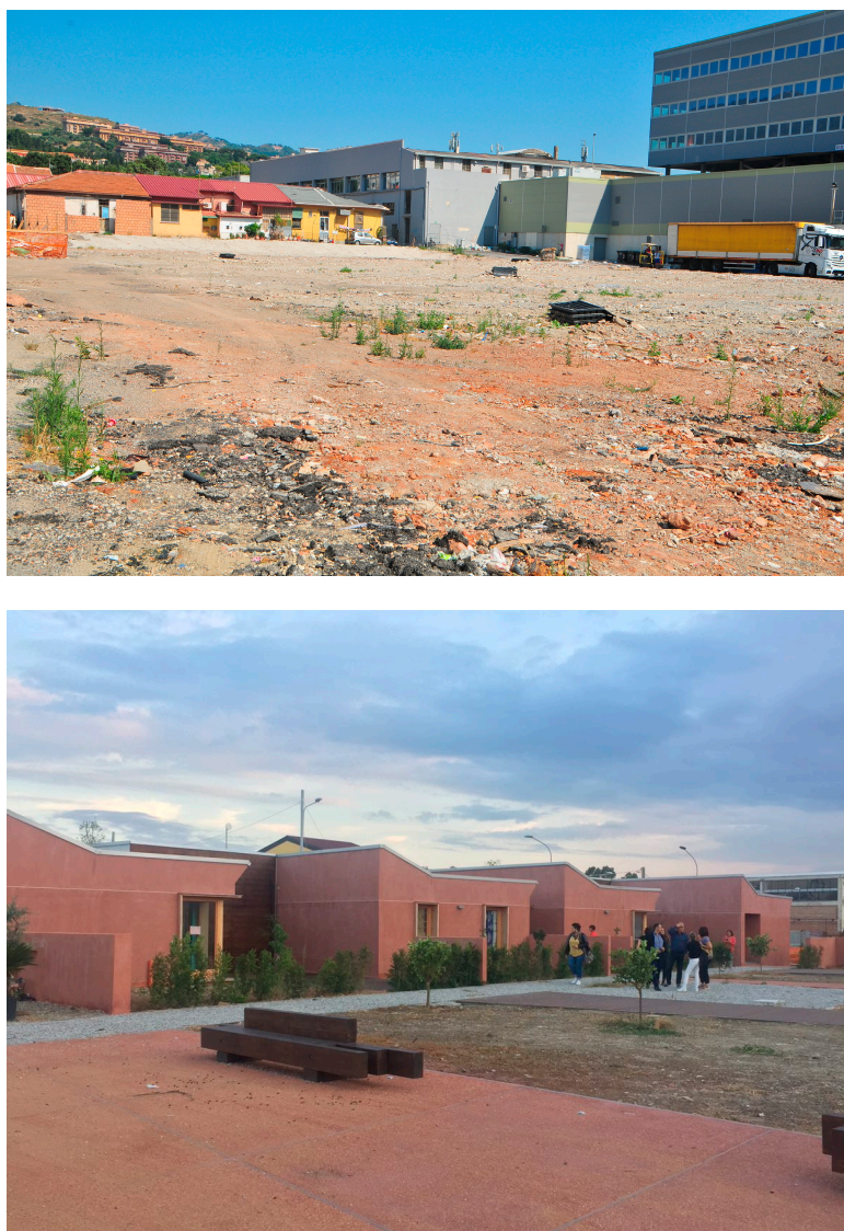
Figure 2. After—Fondo Saccà after the demolition of the slums for the eco-condominium in 2022.
