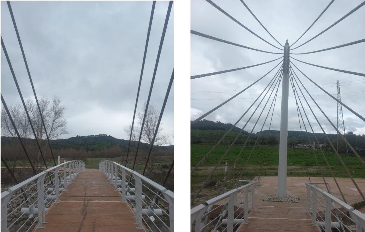
Figure 3.4 - Example of a pedestrian bridge.
