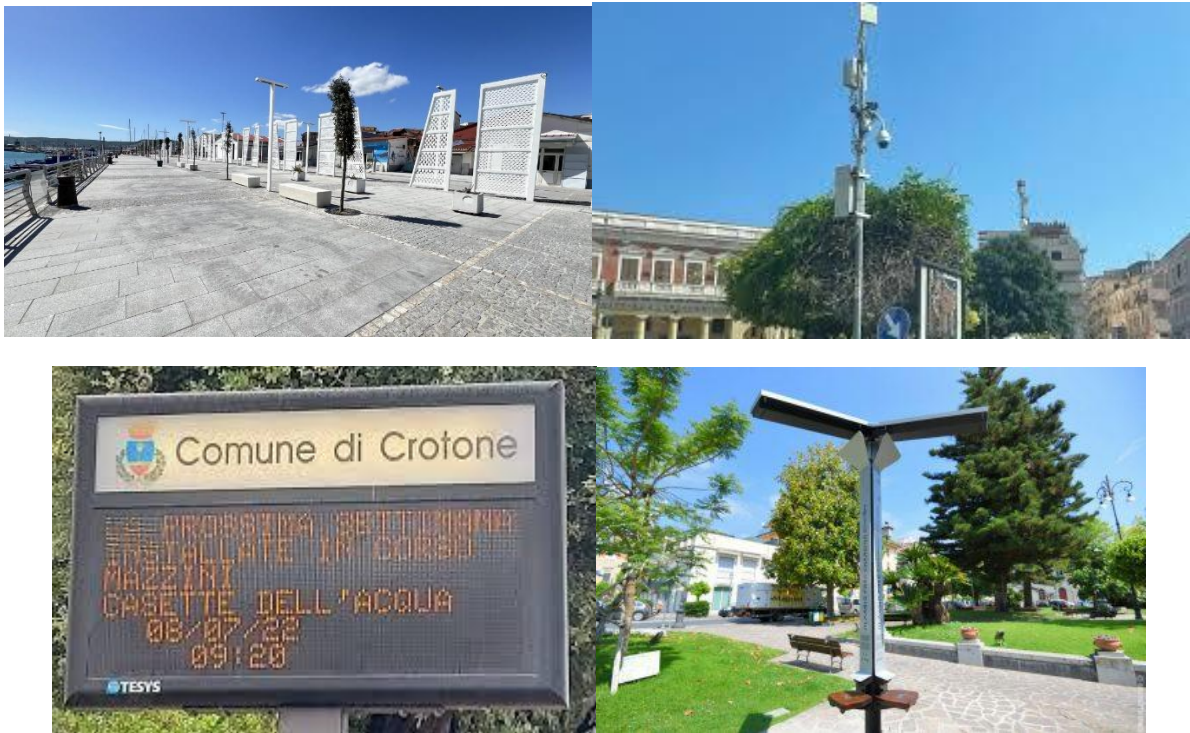
Figure 3.12 - Examples of lighting, urban furniture, video surveillance, communication and charging.
