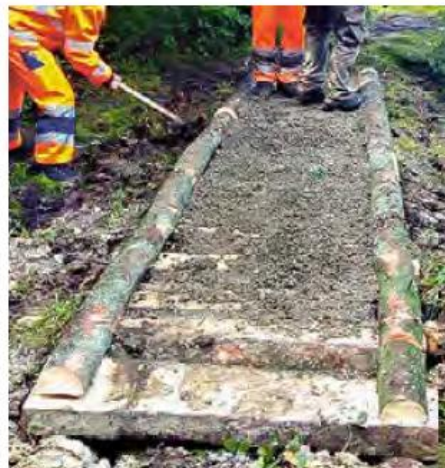
Figure 8.4 - Boardwalk covering with soil and crushed stone.
