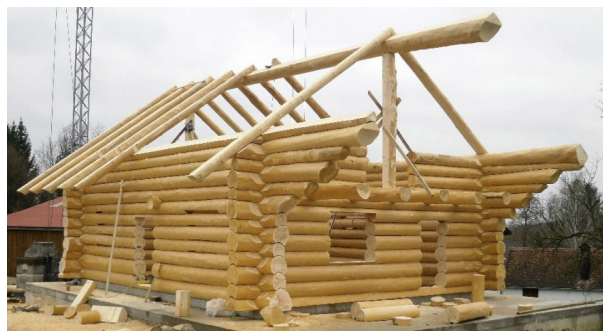
Casa realizzata con sistema blockbau. https://lodge-log-home.com/en/log-frame-houses/
