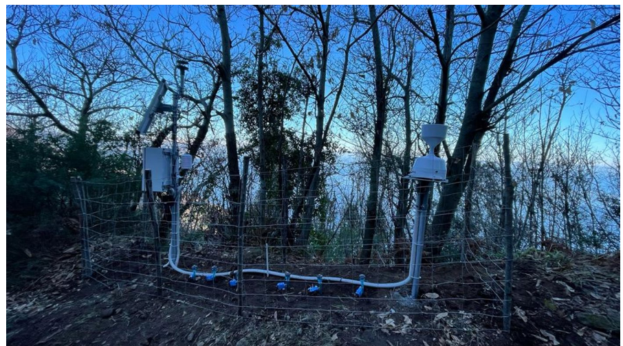
Fig. 4 Monitoring Station N. 1
