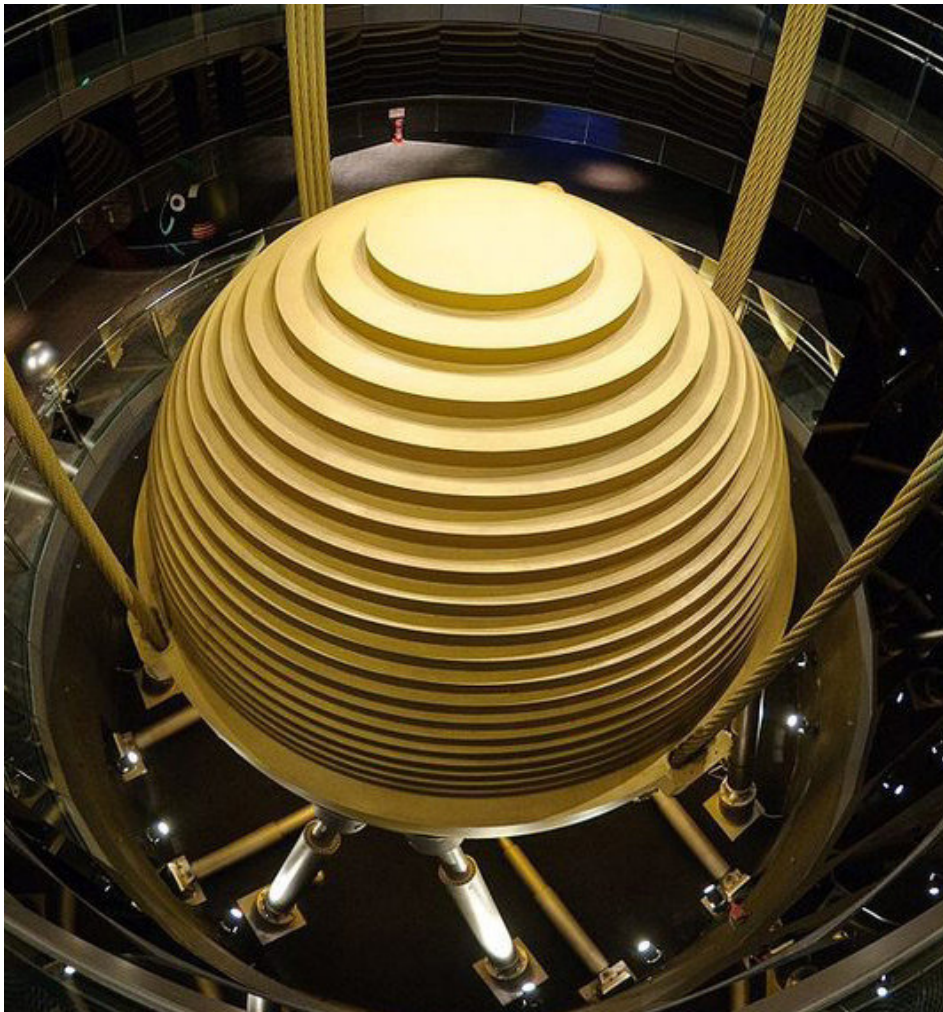
Fig. 6. Tuned Mass Damper of Taipei 101 – Taipei City, Taiwan - Atlas Obscura
