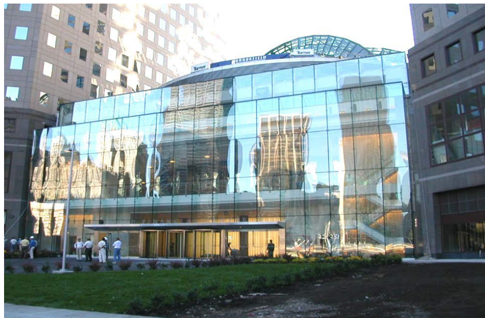
Fig. 1.1 Winter Garden, World Trade Center (Reconstructed). Courtesy of Thornton Tomasetti. Fonte: McFarquhar, D., 2012.
