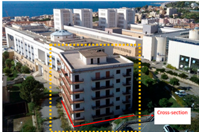
Figure 1. Localization and general view of the case study RC building in Reggio Calabria (Italy).
