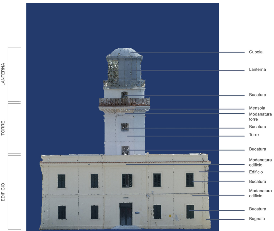
Fig. 13. The Capo Colonna lighthouse: decomposition into macro and micro variables. Fig. 14. The Punta Alice lighthouse: decomposition into macro and micro variables.
