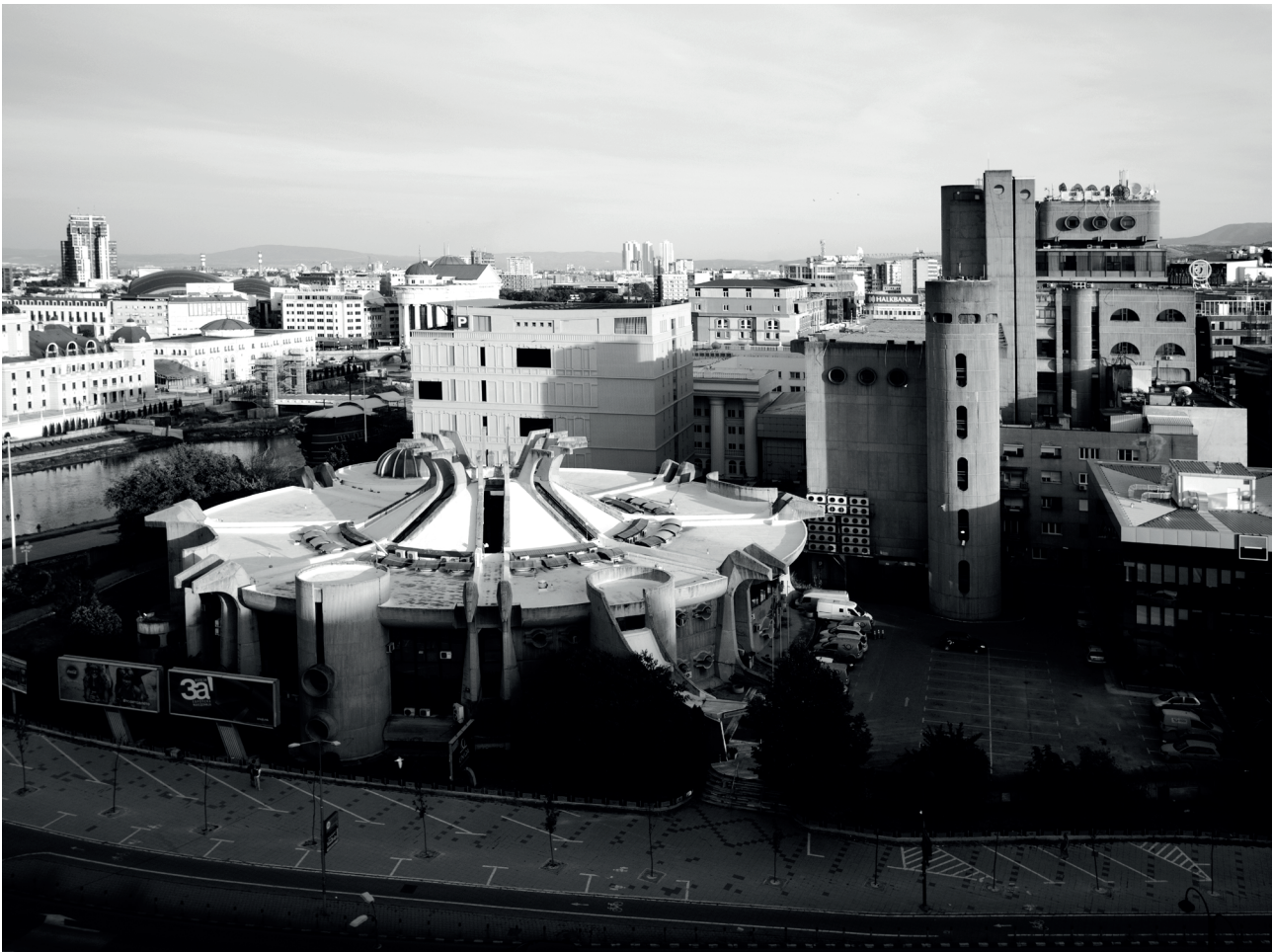
Fig. 4 Janko Konstantinov, Telecommunications Center (1972-1981).
