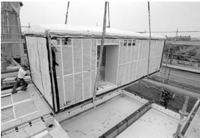
Figure 1. IKEAS' Boklok house installation.
