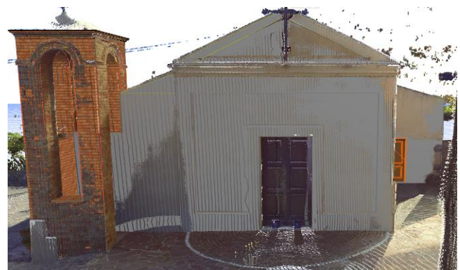
Figure 7. overlap between BIM and Dense Cloud
