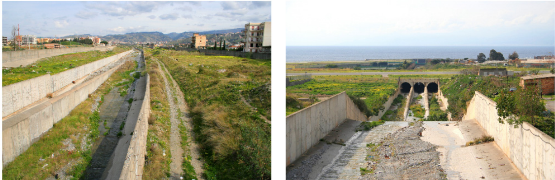
Fig. 3. Channelized reach in urban area with marginal areas in the surroundings.
