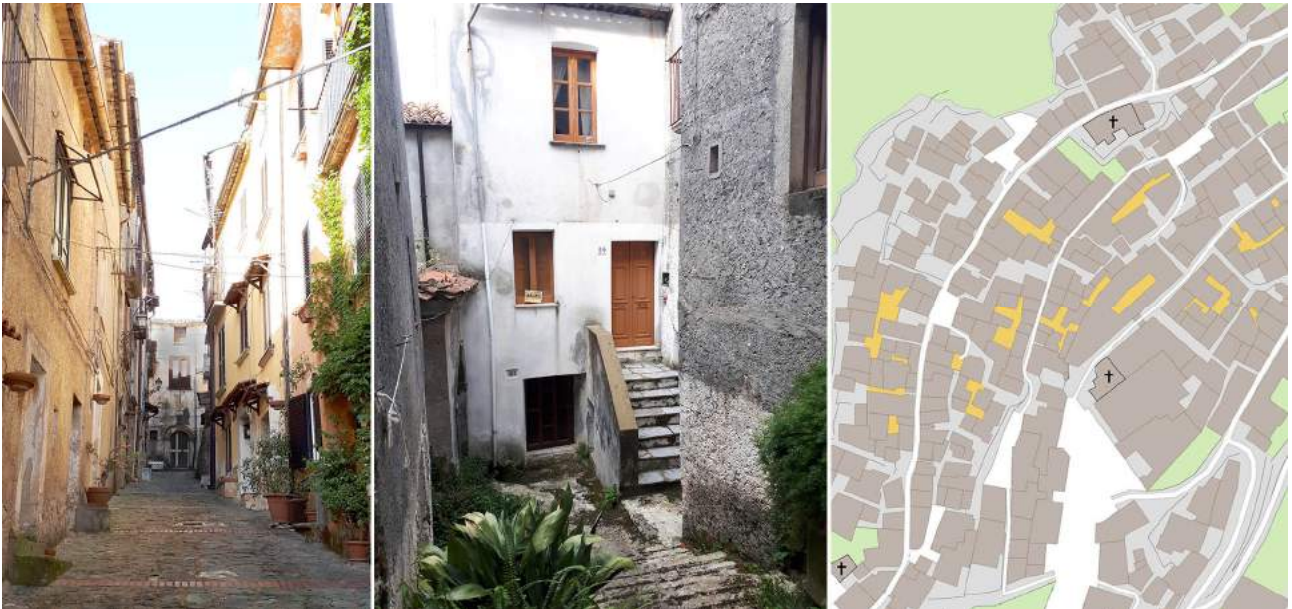
Fig. A1.13 – from left ) A long cul-de-sac in Cerisano, and in Aieta; enclosed, and partially opened courtyards in Santa Severina. Photos by Guglielmo Minervino
