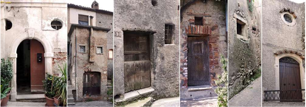
Fig. 4.25 – Examples of openings for natural light in Cosenza, Civita (the two small window open internally inside a fireplace occupying the whole room, with the chimney in the middle), Aieta, Carolei, Mendicino, and Zagarise. Photos by Guglielmo Minervino
