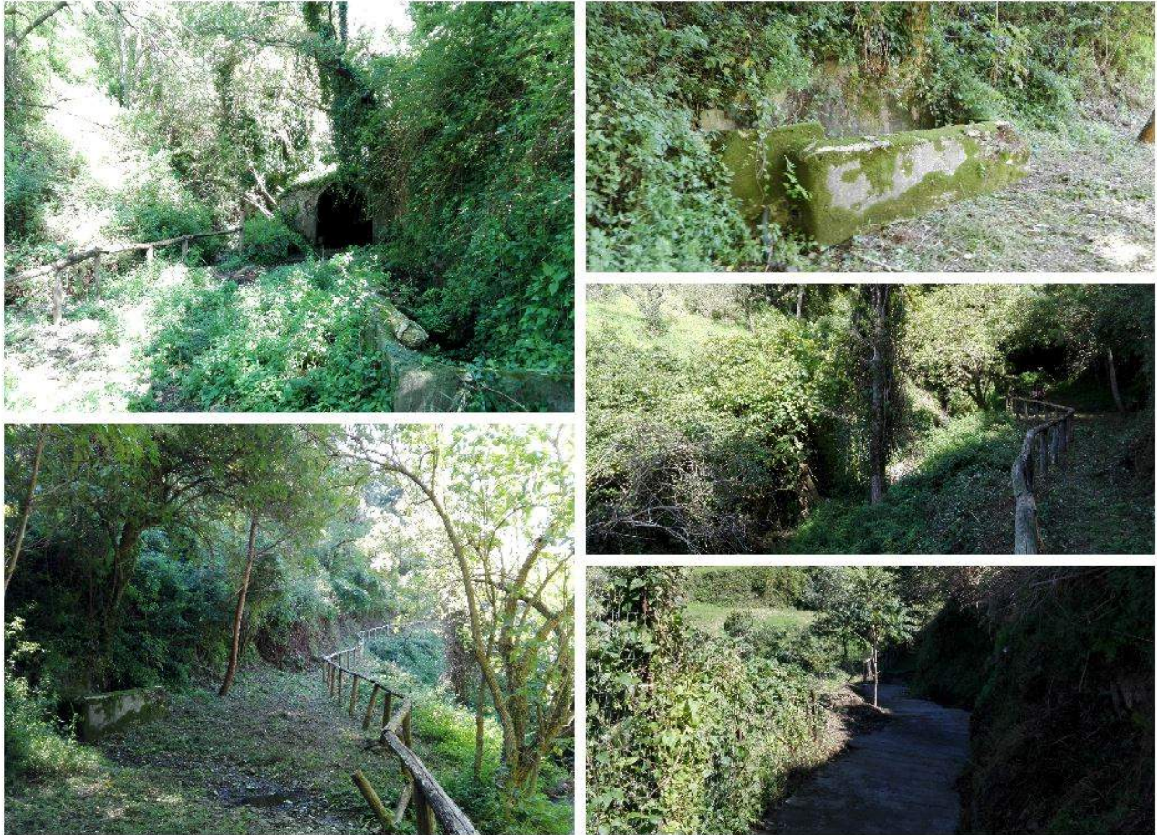
Fig. A6.2 – The wash-house and its surrounding before the intervention.
