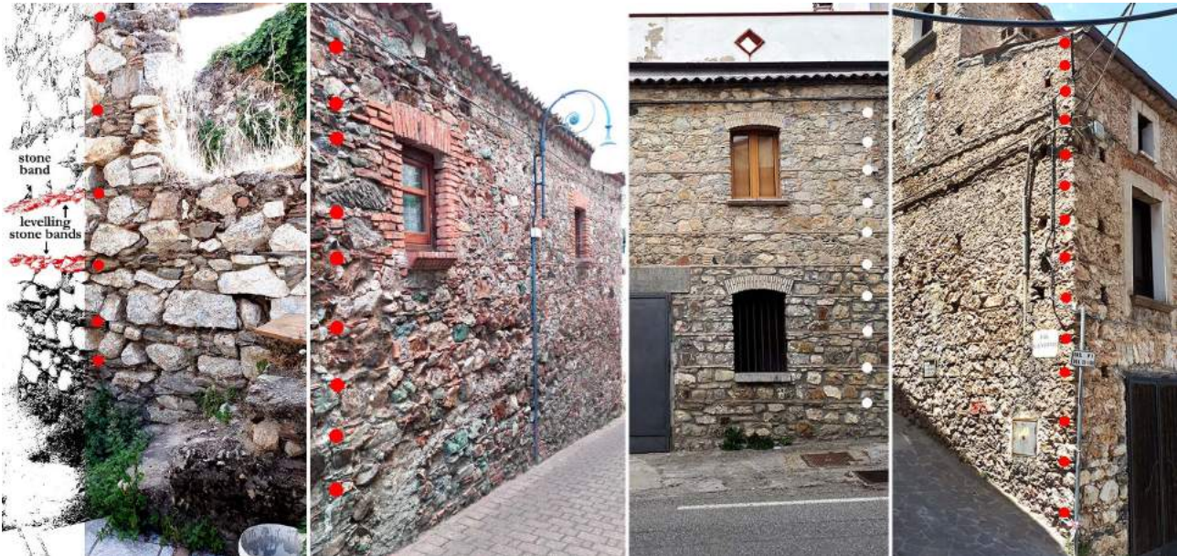
Fig. A1.21 – Examples of walls built with the techniques of alternate bands. From the left in Galliciano, Cerzeto, Cerchiaro di Calabria, San Donato di Ninea. Photos by Guglielmo Minervino
