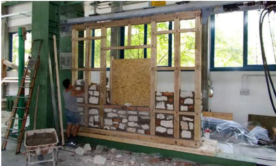
Fig. A1.35 – Building activity of the housing wall section used for the experiment. Photo from
