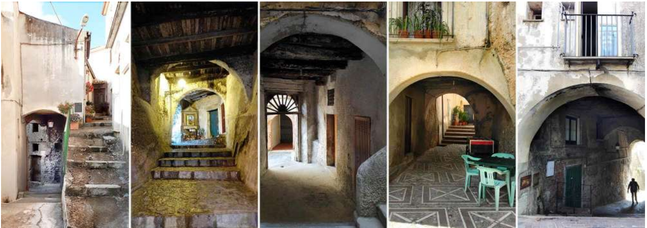
Fig. 4.16 – Examples of Sabat with underneath walkways, from the left in Aieta, Scalea, Mendicino, Cosenza, San Marco Argentano. Photos and drawings by Guglielmo Minervino
