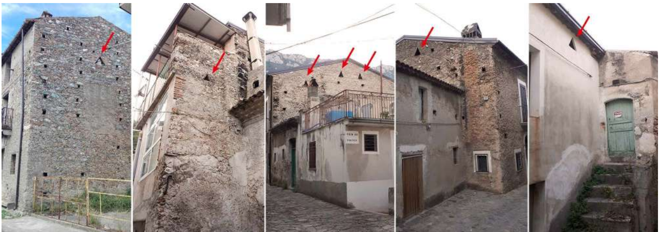
Fig. 4.22 – Pagamuro on walls in Cerzeto (first from the left), and Civita (second to fifth). Photos by Guglielmo Minervino
