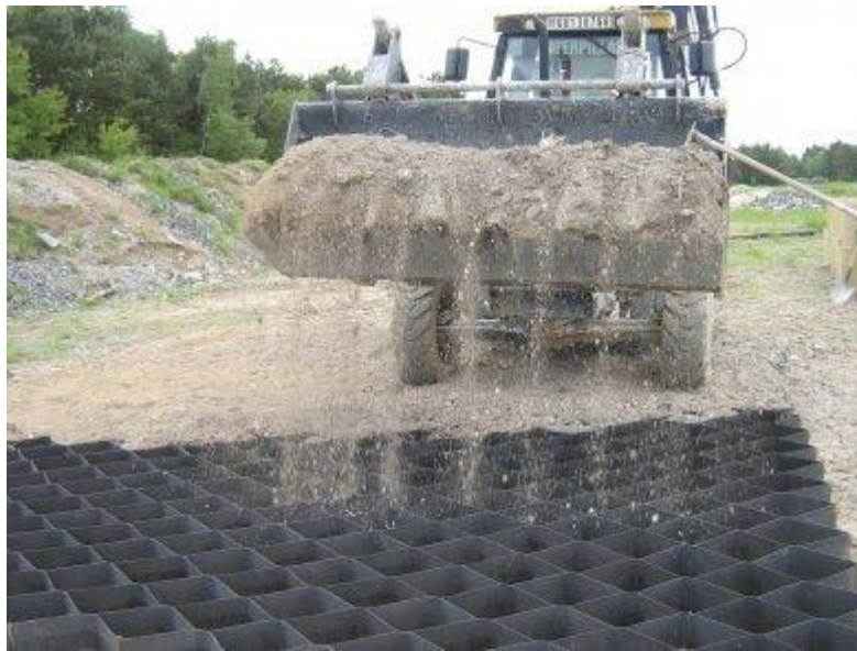
Figure 2.5 Geocells in road application
