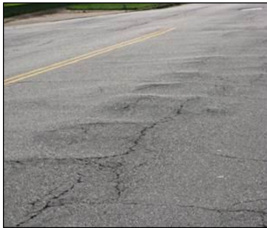
Figure 1.10 Corrugations in asphalt layer
