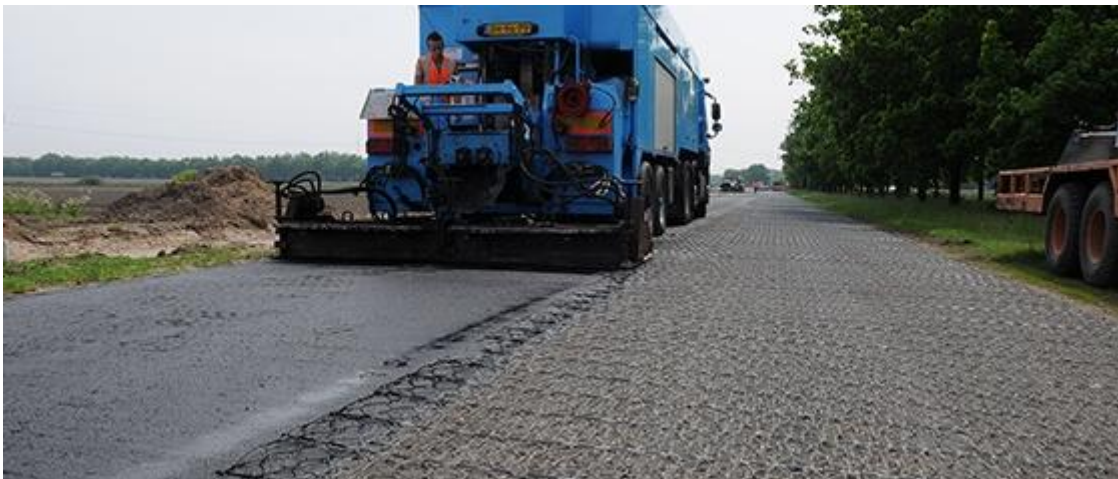
Figure 2.14 Geosynthetic installation in asphalt layer
