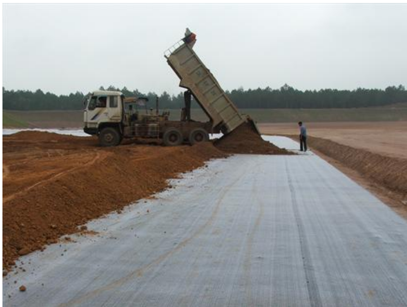
Figure 2.1 Geotextile in road application
