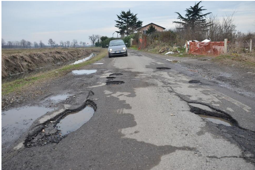
Figure 1.12 Pothole distress
