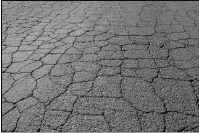
Figure 1.2 Fatigue cracking
