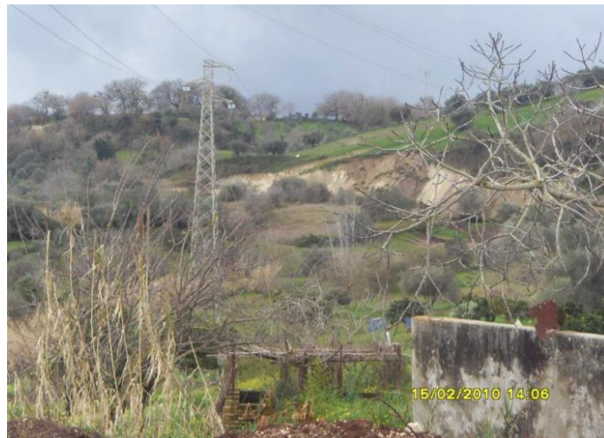
Fig.4.12 d) 2.06pm: pre-existing scarp on the evaporitic limestone gains further at 270 m asl (Pantano locality)
