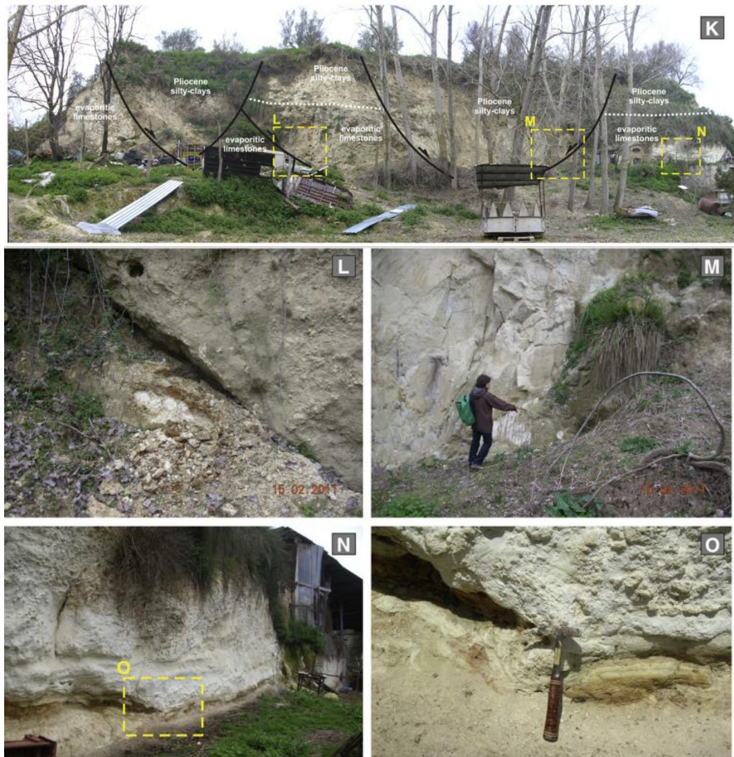
Fig.4.15k-o - Lower sector: K) panoramic view of the trenches, typical of a translational sliding, that caused the spreading of the limestone bank and the sinking of the overlying M) Pliocene deposits (N) decimetric brownish-red and green laminated marl layer, interbedded within the evaporitic limestone, and showing evidence of ductile deformation (O) with a folding that could have been caused by a translational movement of the overlying limestone bank (from Borrelli et al., 2014).
