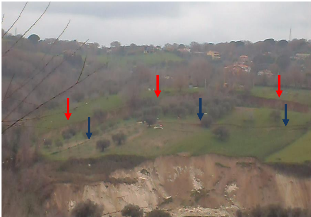
Fig.4.12 f) 4.24pm: main scarp (red arrows) at 300 m asl and secondary scarp formation (blue arrows) at 285 m asl
