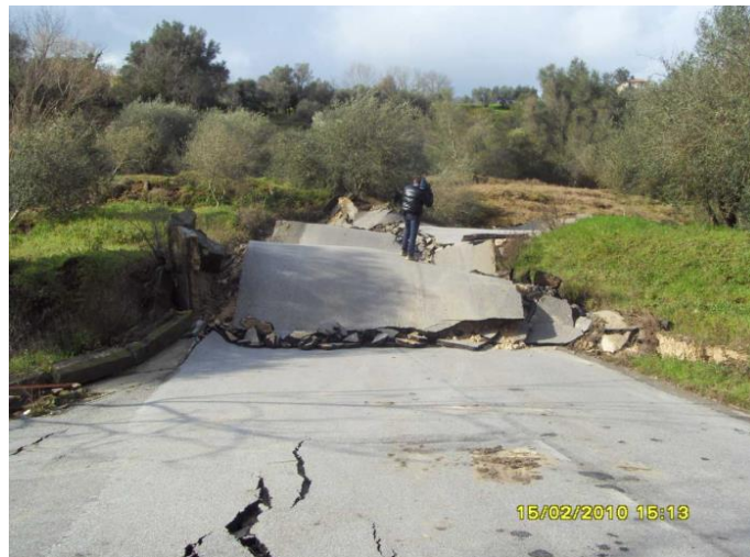
Fig.4.12 c) 3.15pm: deformations on the road S.P. 55 Filogaso-Maierato (Bosco locality)
