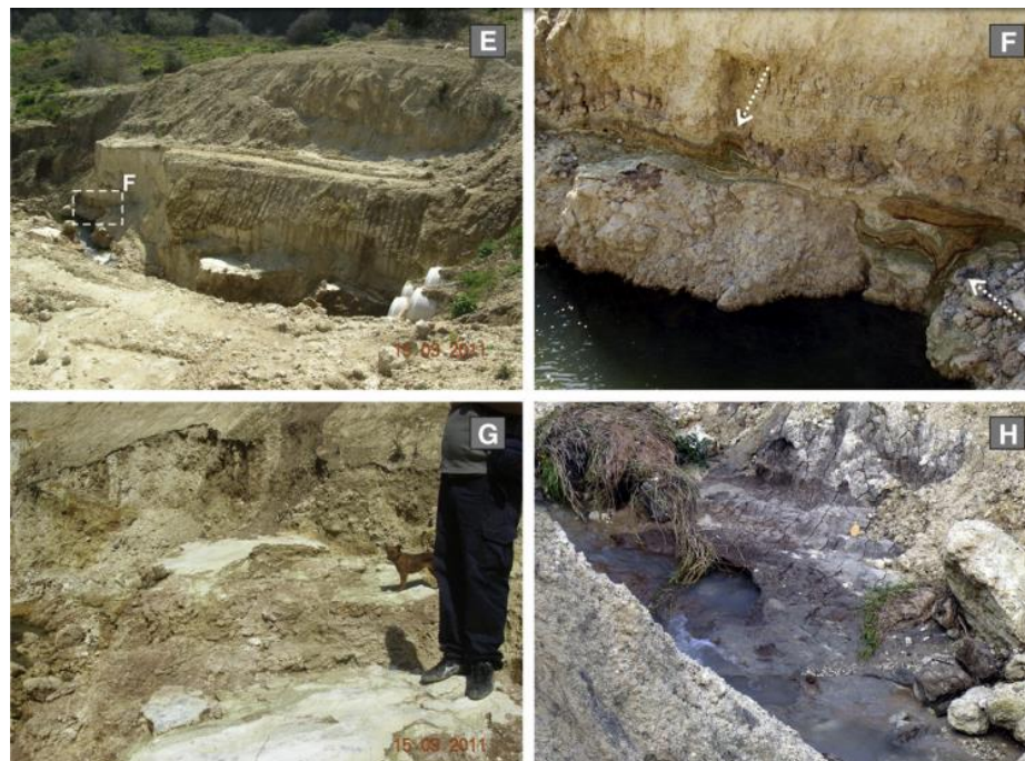
Fig.4.15e-h - Intermediate sector : (E) Very large rock block of evaporitic limestone, little deformed, translated downstream; (F) laminated marl strata, interbedded inside the evaporitic limestone, (G) secondary sliding surfaces exposed on the remnant marl strata; (H) toe of the failure surface of the Maierato landslide daylighting (for about 20 m) in the terminal part of the intermediate sector. (from Borrelli et al., 2014)
