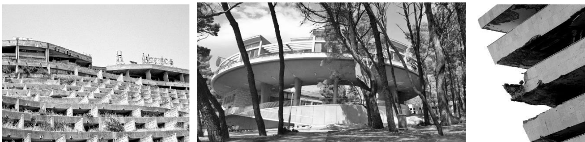
Figure 13. Libertas Hotel in Dubrovnik, Lječilište in Kravice, Kupari Hotel in Župa Dubrovačka (Source: Author)
