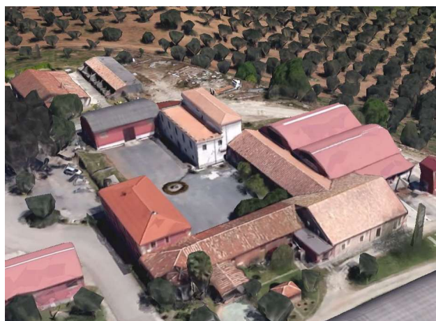
Figure 2. 3D vision of the case study: a historic rural building complex in Calabria.
