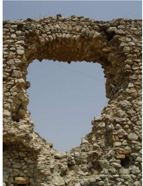
Fig. 4 Belcastro (CZ). The “heart” before the masonry reinforcement.
