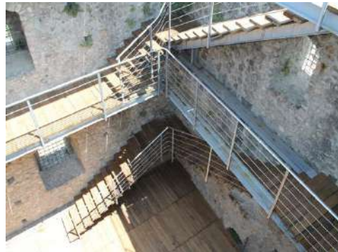
Fig. 3 Belcastro (CZ), the interior part of the Donjon. Ramps and walkways during the construction.
