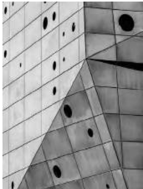
[3] _ Detail _ Roskilde Waste Incineration Plant- Control Room in Denmark by Erick van Egeraat [source: web]
