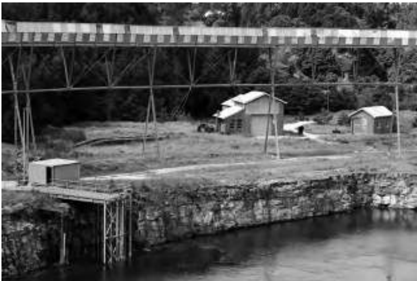
img.1 _ Sites of manufacture - The Brickpit Ringwalk at Sydney Olympic Park, a colourful structure hovering above the sandstone floor of the pit, now filled with water. A wasteland turned into habitat for the endangered Green and Golden Bell frog, as well as an architectural landmark to experience the fragility of nature. Ph: Giamila Quattrone, February 2015.
