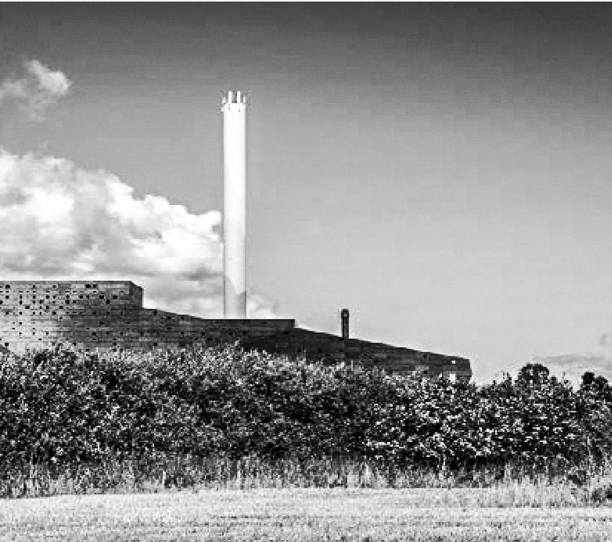
[3] _ Roskilde Waste Incineration Plant-Control Room in Denmark by Erick van Egeraat [source: web]
