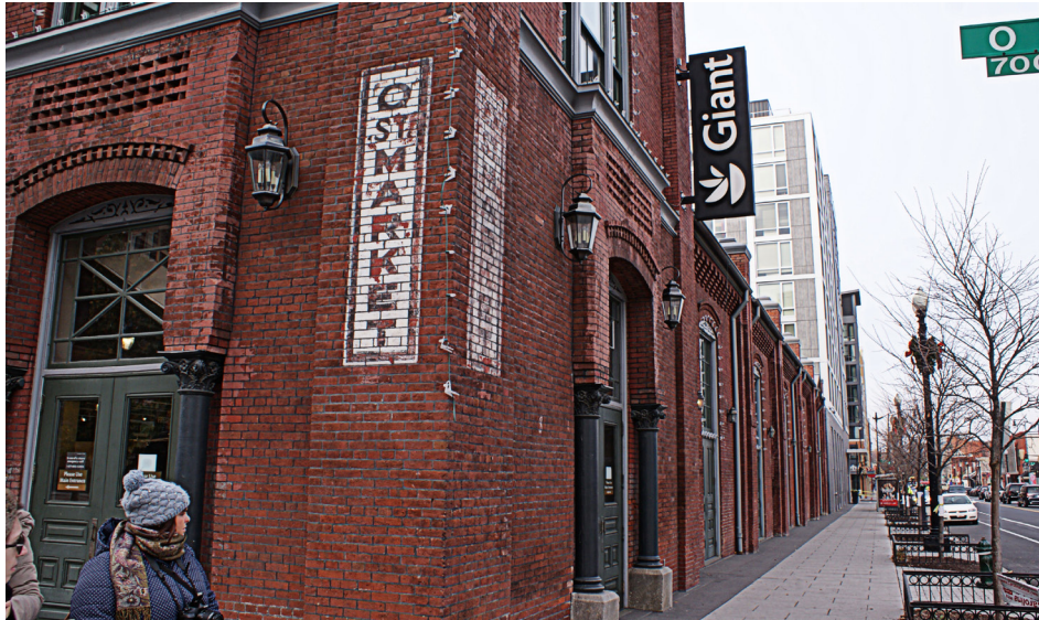
Figure 4 | The Giant Food Supermarket at O Street.
