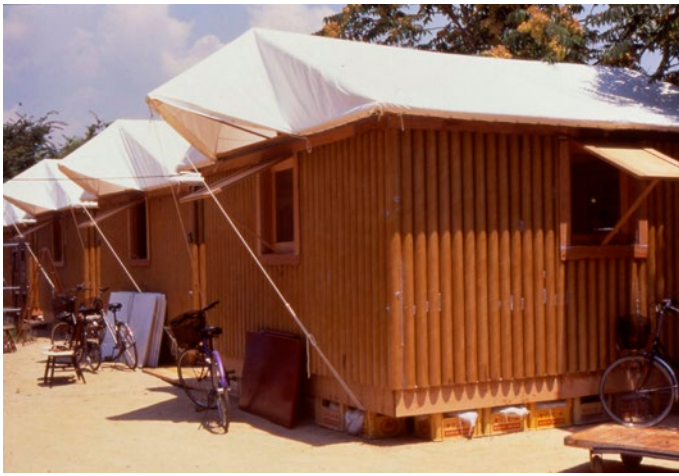
01 | a) Paper Log House, Shigeru Ban Architects - Kobe. Photo Credits by Takanobu Sakuma; b) Paper Log House, Shigeru Ban Architects - Turchia, sezione scala 1:50. Credits DWG: Shigeru Ban Architects a) Paper Log House, Shigeru Ban Architects - Kobe. Photo Credits by Takanobu Sakuma; b) Paper Log House, Shigeru Ban Architects - Turkey, section 1:50. Credits DWG: Shigeru Ban Architects
