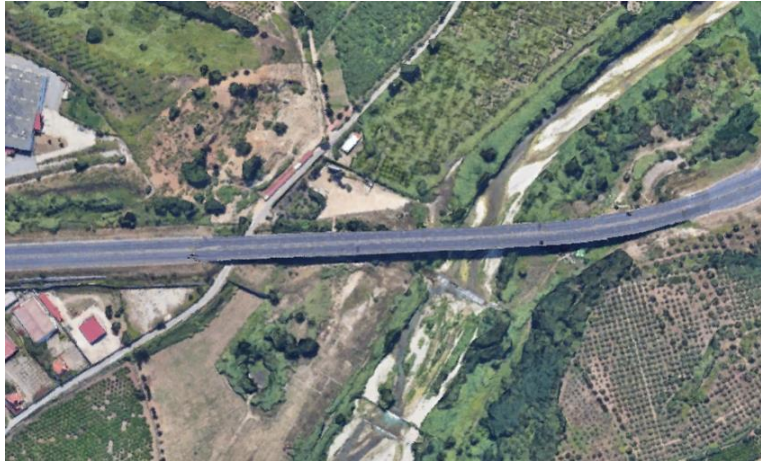
Figura 5.8 - Case Study: Road Bridge in Reggio Calabria (between Palmi and Gioia Tauro) South Italy
