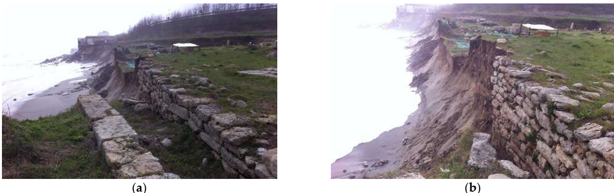
Figure 6. Doric Temple. (a) After the December 2013 storm. (b) After the February 2014 storm.
