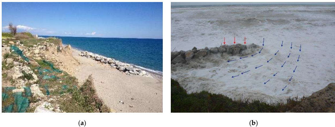
Figure 7. (a) Barrier made in January 2014. (b) Storm of February 2014 (blue arrows) that crosses the barrier (red arrows).
