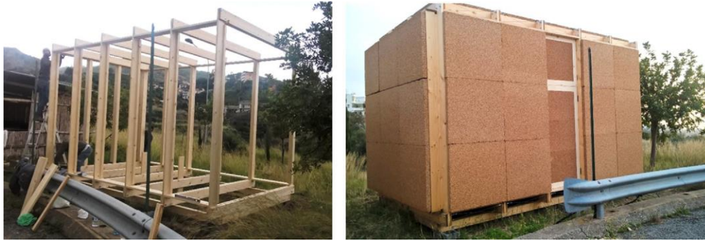
Fig. 6. Construction of the shelter prototype.
