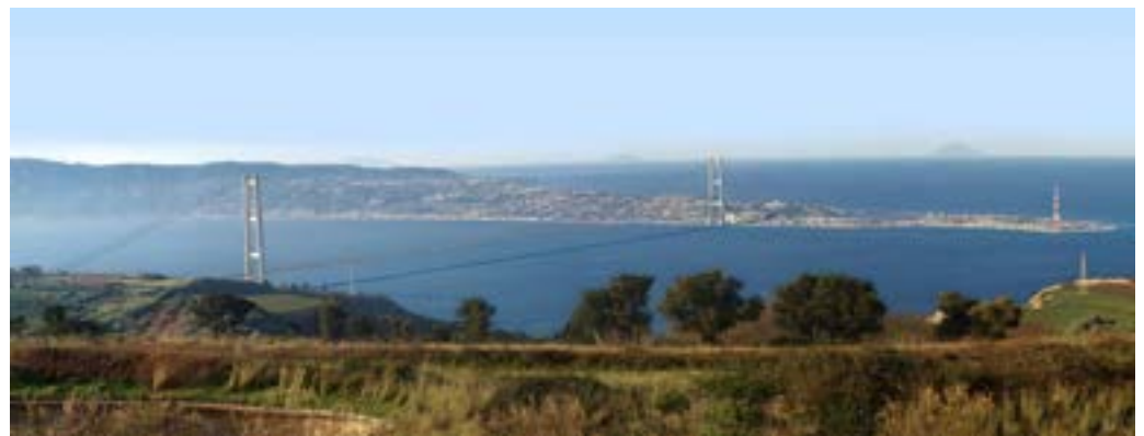
Figure 4. View of the Strait with the Bridge. Credit: Webuild—Stretto di Messina S.p.A.
