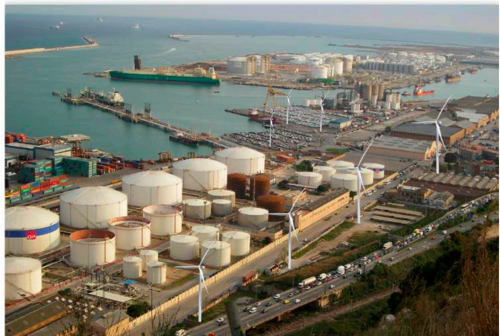
Figure 8. Port infrastructure. Example of an installation hypothesis in a representative scenario through the application of the identified criteria. Criteria adopted: 1: In general, for a set of wind turbines, a more positive image is produced with a small number of large wind turbines instead of
